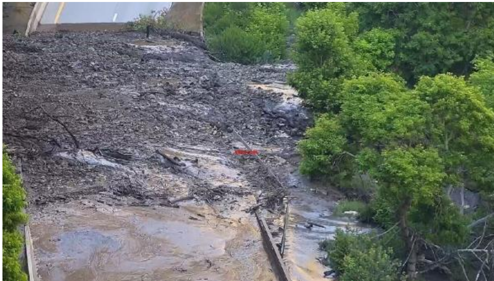
(Fig. 1: Debris Flow Covering Eastbound Lanes of I-70 in Glenwood Canyon) 1
